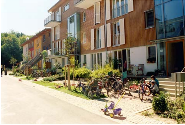
FREIBURG: Instead of giving space to the car, the residential neighbourhood can have much open space provision.
