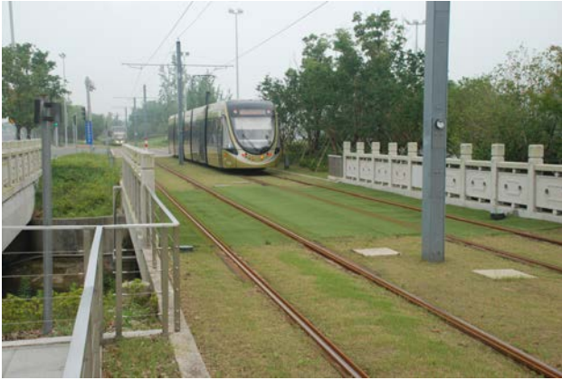
SUZHOU: China may be the context where multiple modes of public transport are most required – and where the new innovations can be developed.
