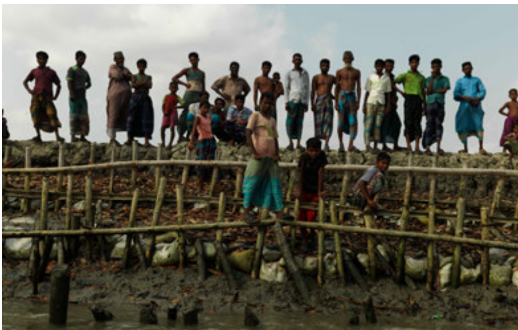
Villagers at Kalabogi village, Bangladesh, stand on a makeshift dike. If this dike breaks over 1,000 homes will be washed away. At high tide the sea is inches away from bursting the bank
